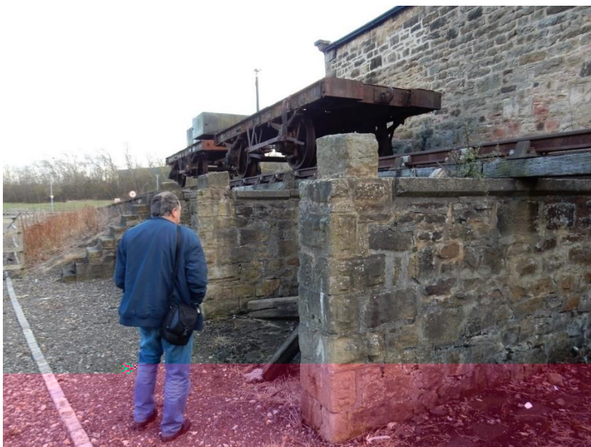
Plate 8. The elevated ramp to the rear for dropping coal into waiting carts for domestic sale, known as being taken to the port for export) (The photo shows Ken Hodgson who is a leading light in raising the profile of heritage)
