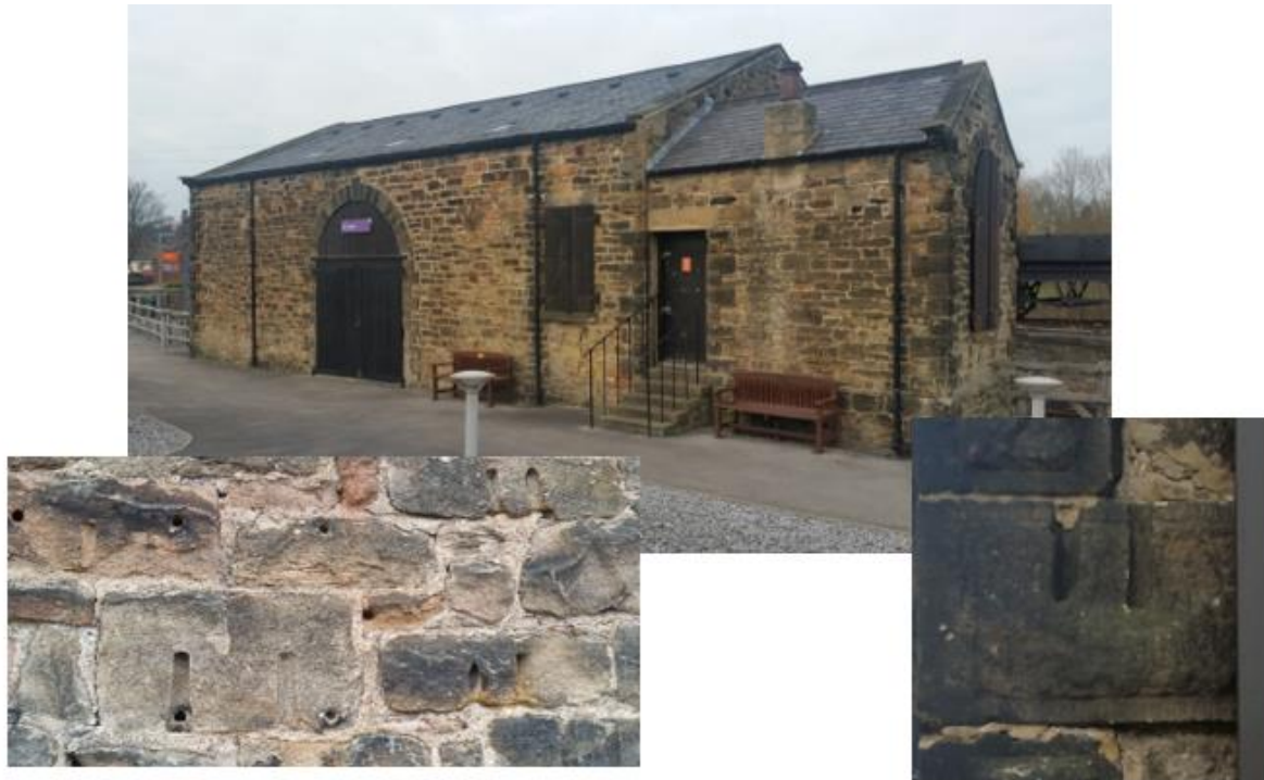
Plate 7. The Goods Shed and detail of reused two hole sleepers in the fabric of the building
