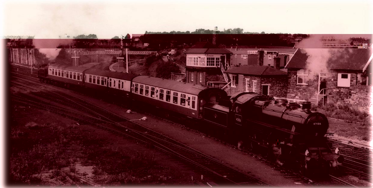
Plate 3. An undated photograph of the signal box and adjacent buildings and the coal drops in the distance in British Railway days
