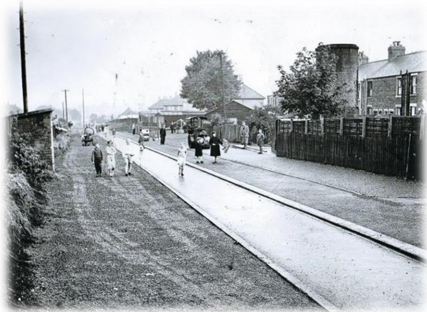
Plate 14. The ventilator shaft (on the right behind the tree) behind Windsor Terrace in 1962 adjacent to the footpath.
